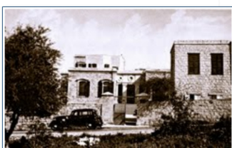
'Abdu'l-Baha's home in Haifa. The extra rooms on the roof were built for Shoghi Effendi in 1923 at the request of the Greatest Holy Leaf.
